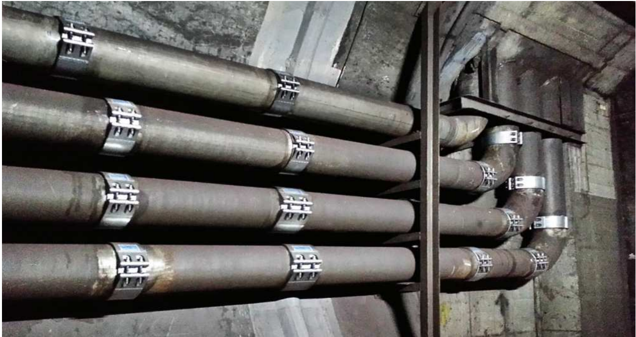
▲ Underground drainage repair(Maintenance) works
