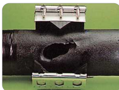
▲ REPAIRING THE PIPES
