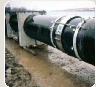
▲ U.S.: nuclear power plant
