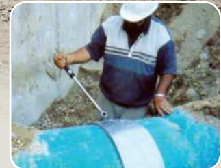
▲ UK: buried water supply pipes
