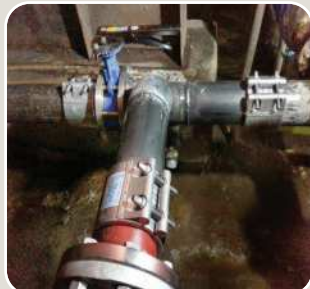
▲ Netherland desalination treatment facilities
