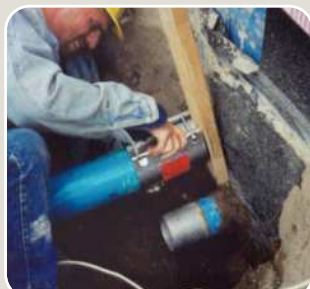
▲ U.S.: sewerage repair work
