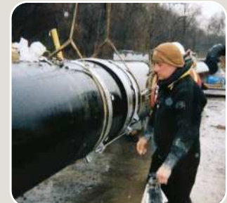
▲ UK: district heating work
