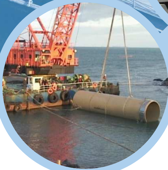
Installation of ocean bed blocks
