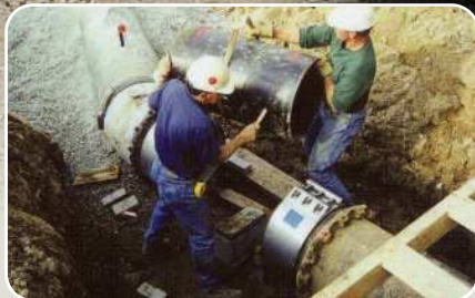
▲ Repair work for pipes replaced underground
