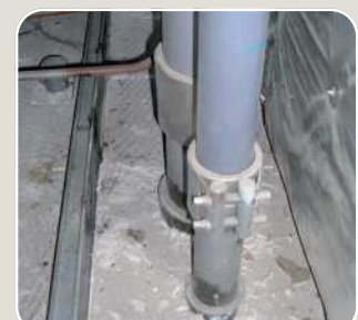
▲ PVC + Steel Pipe Connection
